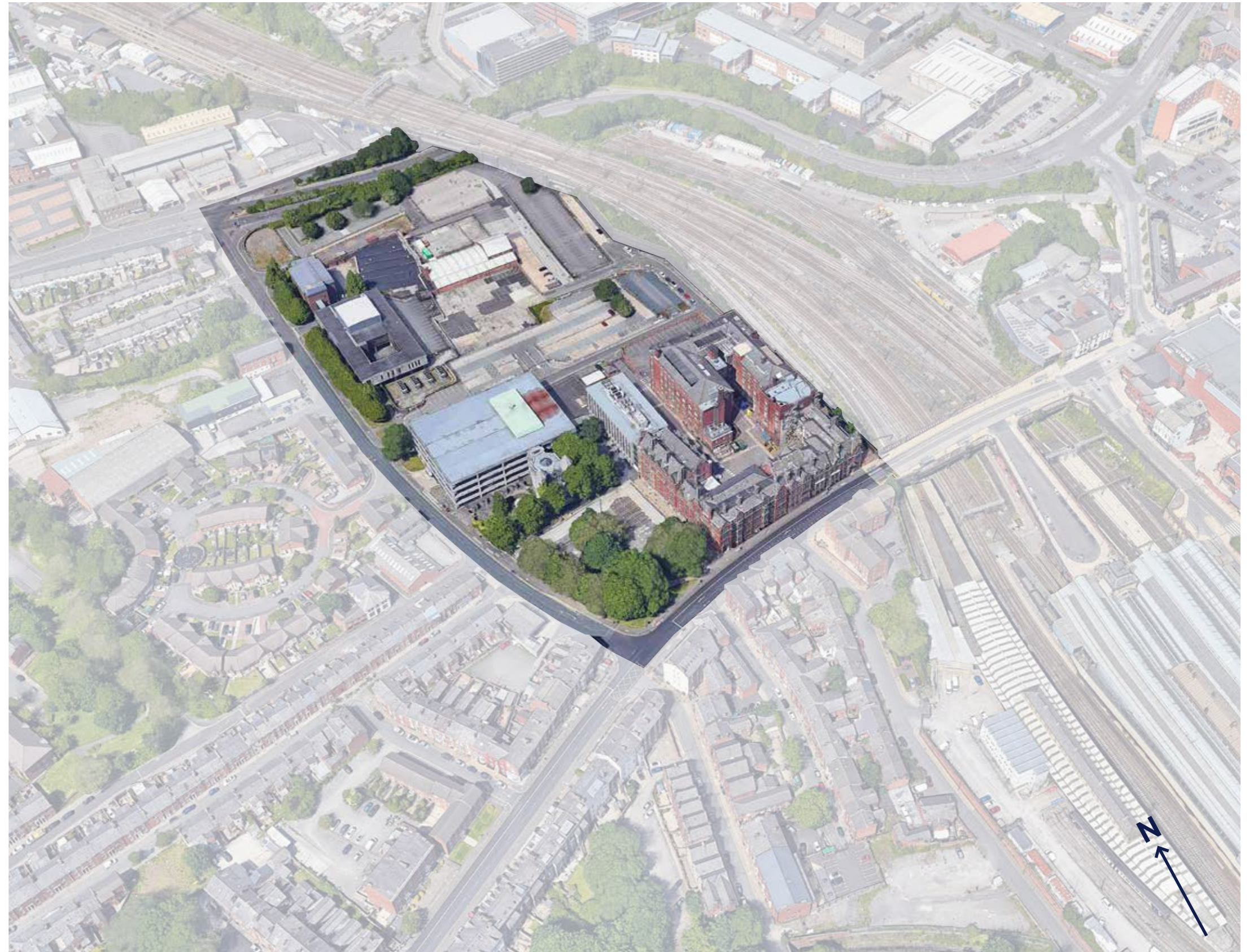
Figure 7.4.1: County Hill Scope Area
