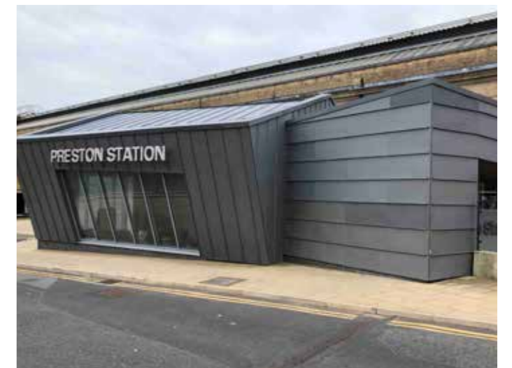
Butler Street entrances to Preston Station
