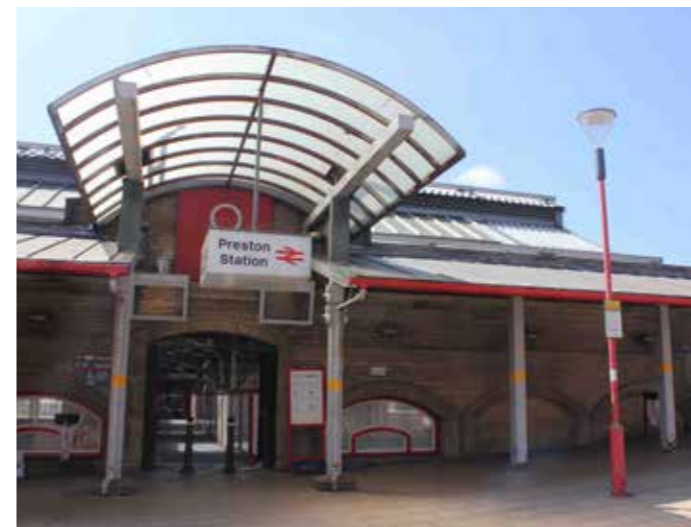
Butler Street entrances to Preston Station
