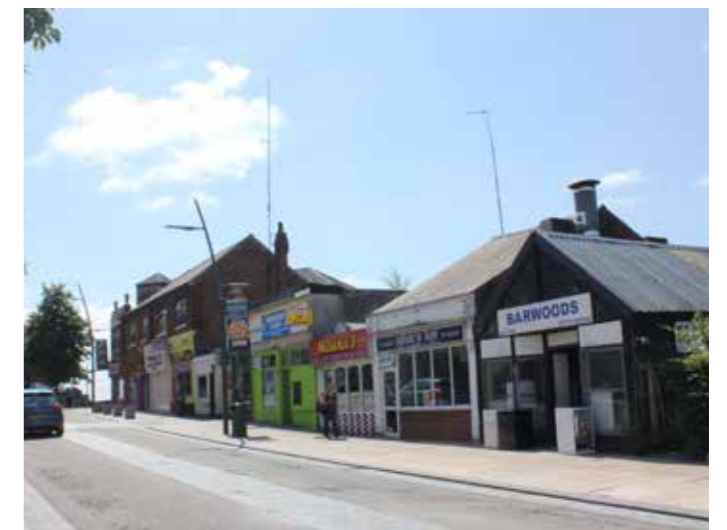
Commercial premises on Corporation St
